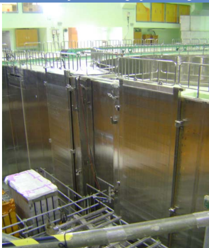
Nuclear power storage pool lining
